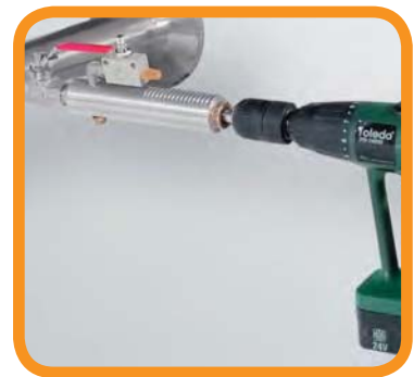
Drilling under pressure
